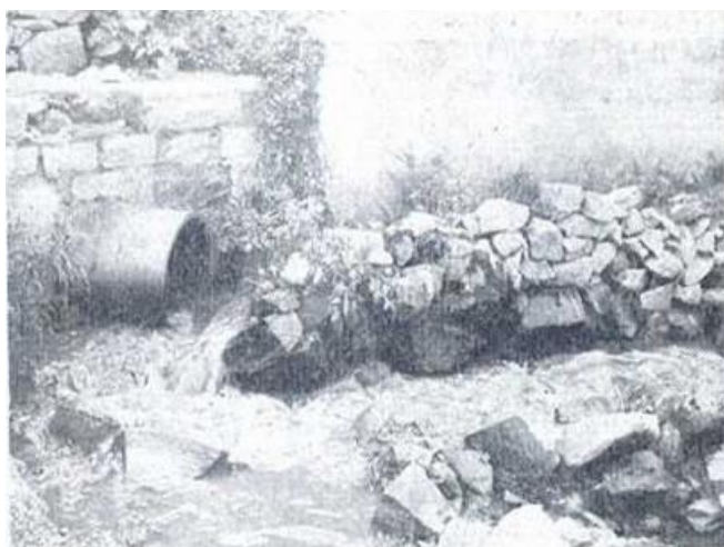
First zone: Discharge of raw sewage over rocks. Preliminary changes leading to clarification and oxygenation.
